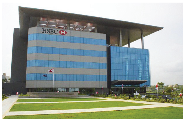
HSBC's GLT in Pune, India has installed technologies that reduce carbon dioxide emissions by 700 tonnes per year.
