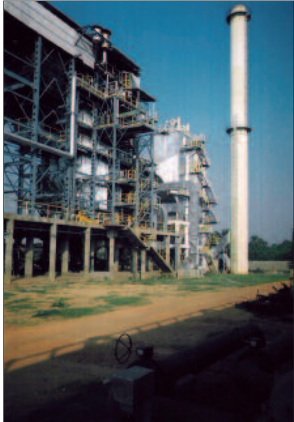
The Vensa Biotek biomass co-generation facility in Andhra Pradesh, India.
